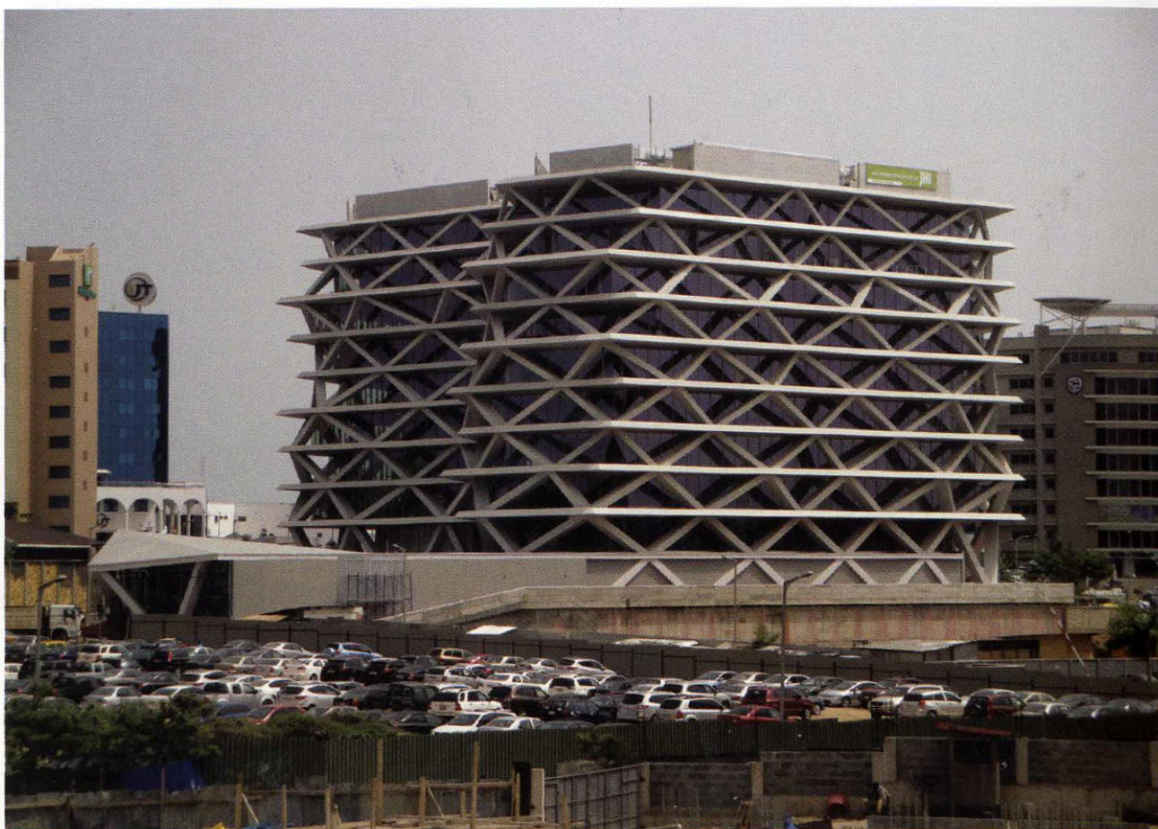
One Airport Square is Ghana's first building to be constructed on seismic isolators.
