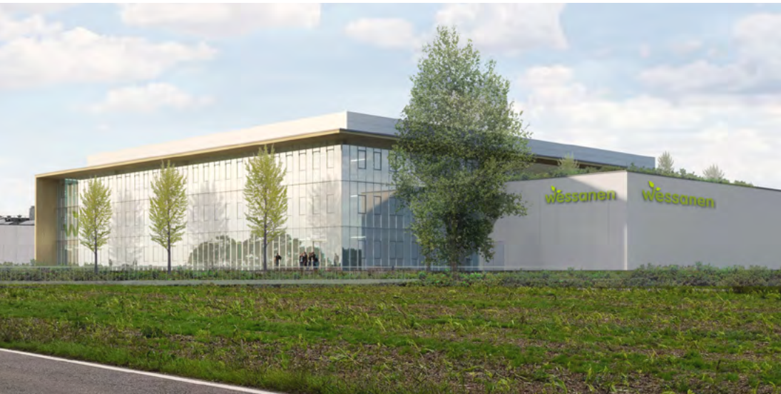
ABAFOODS ENLARGEMENT OF THE PLANT Badia Polesine, Italy
