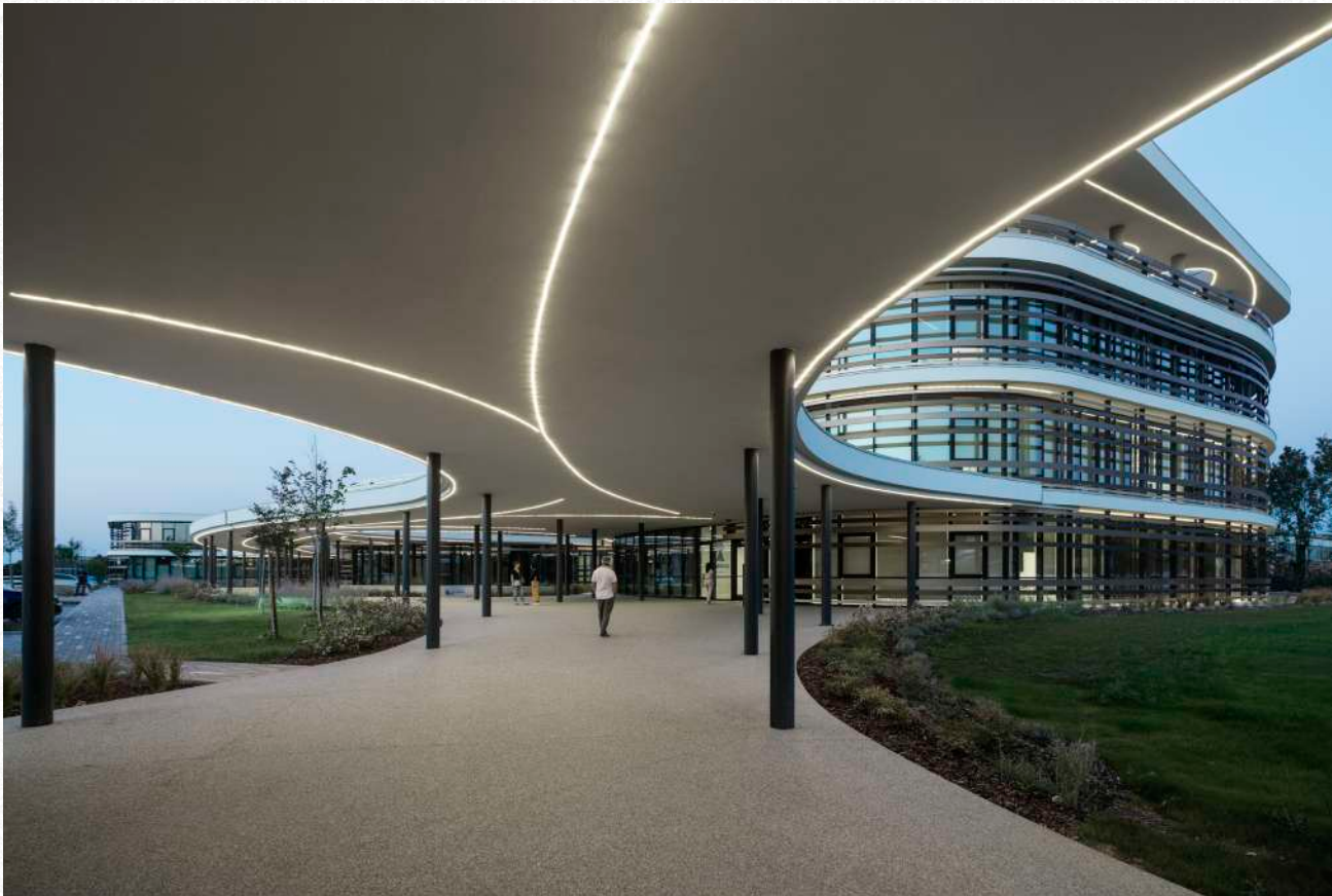
Management Center space'TENGO Coop Reno, Bologna
