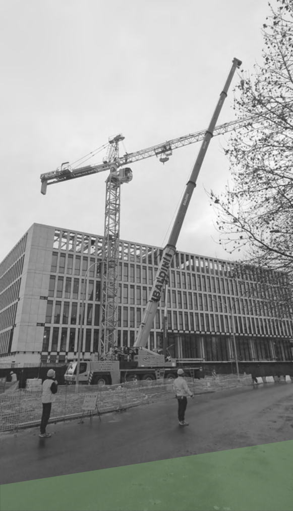
Crif21 construction site, Bologna.
