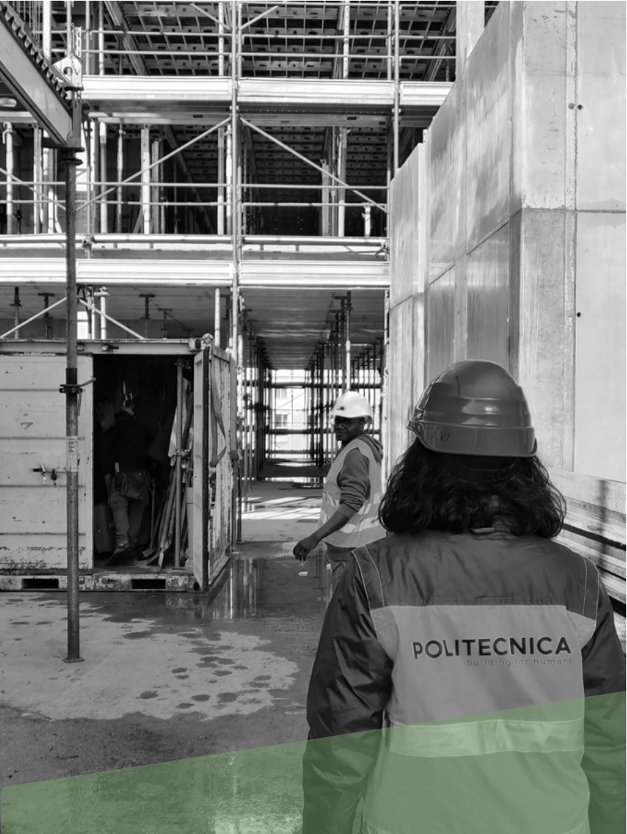
Unimib U10 Logos construction site, Milan.
